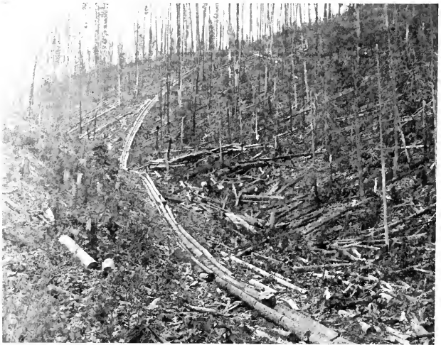
FIG. 84. — A Two-pole Running Log Slide. Idaho.
